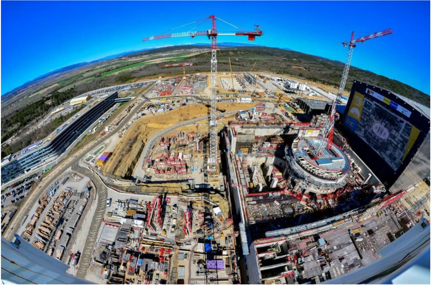
Slika 1.2: Tokamak kompleks (preuzeto s https://www.iter.org/construction/tkmcomplex )
